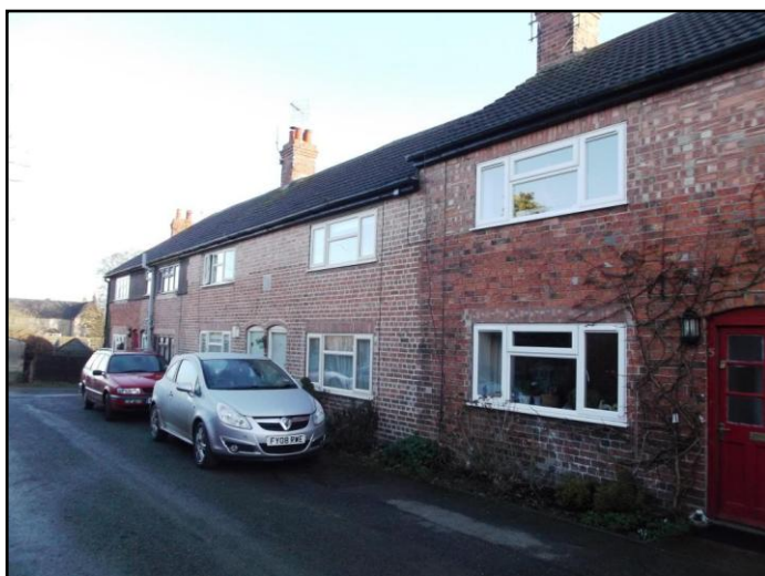
Fig. 15 UPVC windows at Back Row have undermined the historic character of the terrace.
