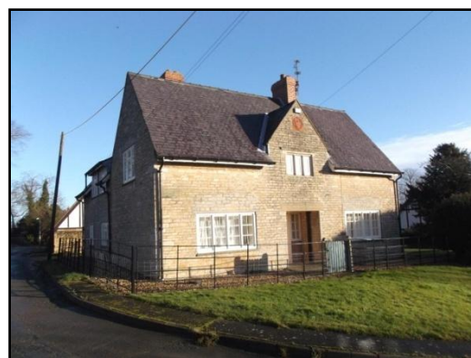
Fig.13 Church Farm, located opposite The Green, Church Street. It has the coat of arms of the Easton Estate above the door on the central gable.
