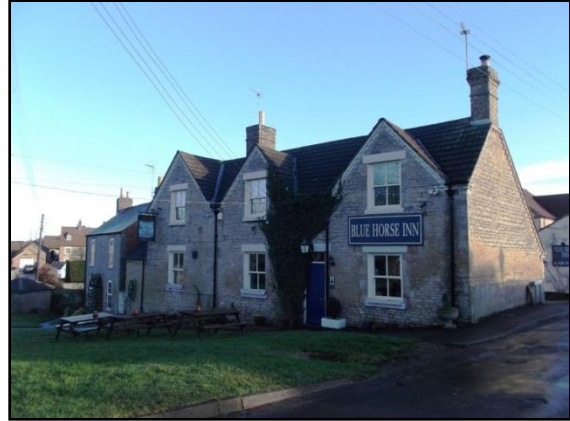
Fig.2 The Blue Horse Inn. One of a number of important buildings of local significance that enclose The Square and contribute towards a cohesive character.
